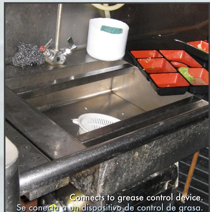
Connects to grease control device.
